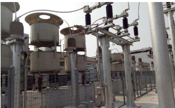
4# LF Refining Furnace Project of Xinyu Iron and Steel TSVC-35kV-27000kvar/27000kvar
