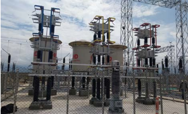
Columbia union project shunt capacitor installation project TBB115-5000/446.3-BLW
