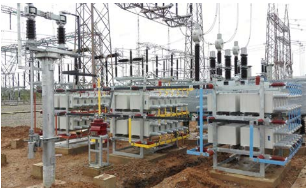
Zambia State Grid Corporation 11 kV Shunt Capacitor Installation project TBB11-30000/430-BLW
