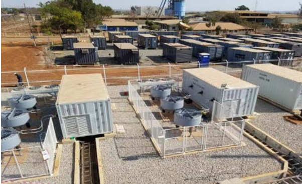
Tanzania Voltage drop compensation project for Buly Gold Mine project ZTSVG-C15/6.6-O-W
