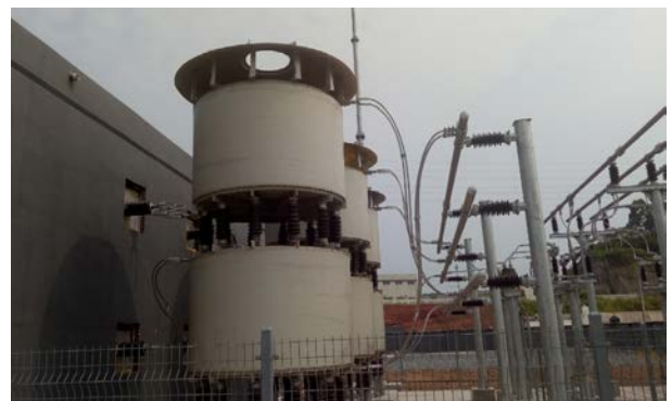
Tangshan Rixin Energy Co., Ltd Submerged arc furnace project TSVC-35kV-25000kvar/20000kvar
