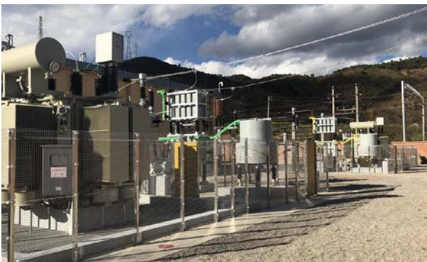
Inner Mongolia Shuangxin Chemical Engineering Project MSVC-35kV-20000kvar/20000kvar
