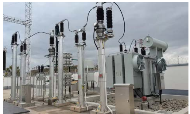
Yunnan Qujing Xiaoxin Street Substation Project MSVC-35kV-14400kvar/9600kvar
