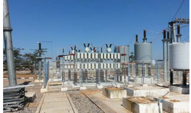
Zambia State Grid Corporation 66kV shunt capacitor installation project TBB66-30000/489-BLW
