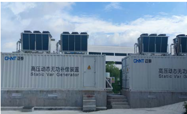
High-power test Compensation project of Dekai Test Center ZTSVG-C50/10-O-W
