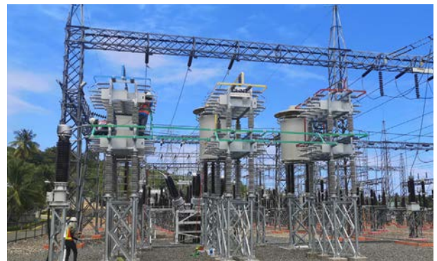
Philippines 138 kV Outdoor Capacitor Complete Installation Project TBB138-20000/496-BLW
